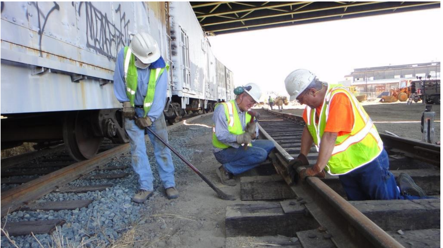
Mike M. “nips” the tie. Steve sets the spike ready to hand the hammer to John so he can do the same on the other side
