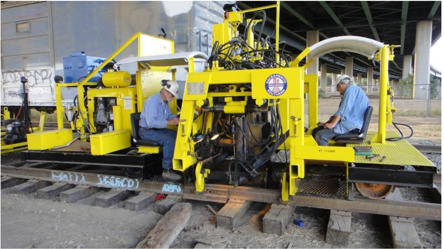
With the Super "B" repaired, Alan, and Mike H. (on the other side) operate the spiker-rams while Fred feeds spikes into the chutes
