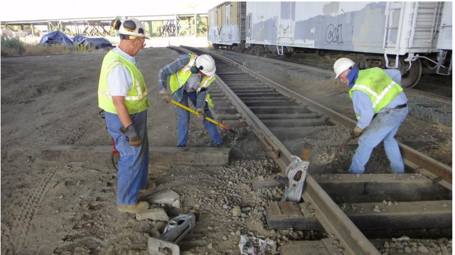
Clem stands ready with tie-tongs to move the tie as Steve and Mike M. dig to make some room for it under a joint
