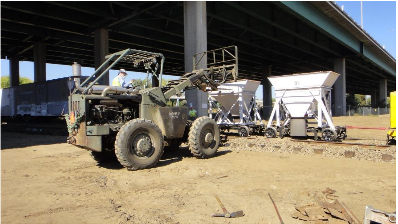
Mike M. on Big Green tries to use the all-terrain fork-lift to shake the junk loose inside the hopper
