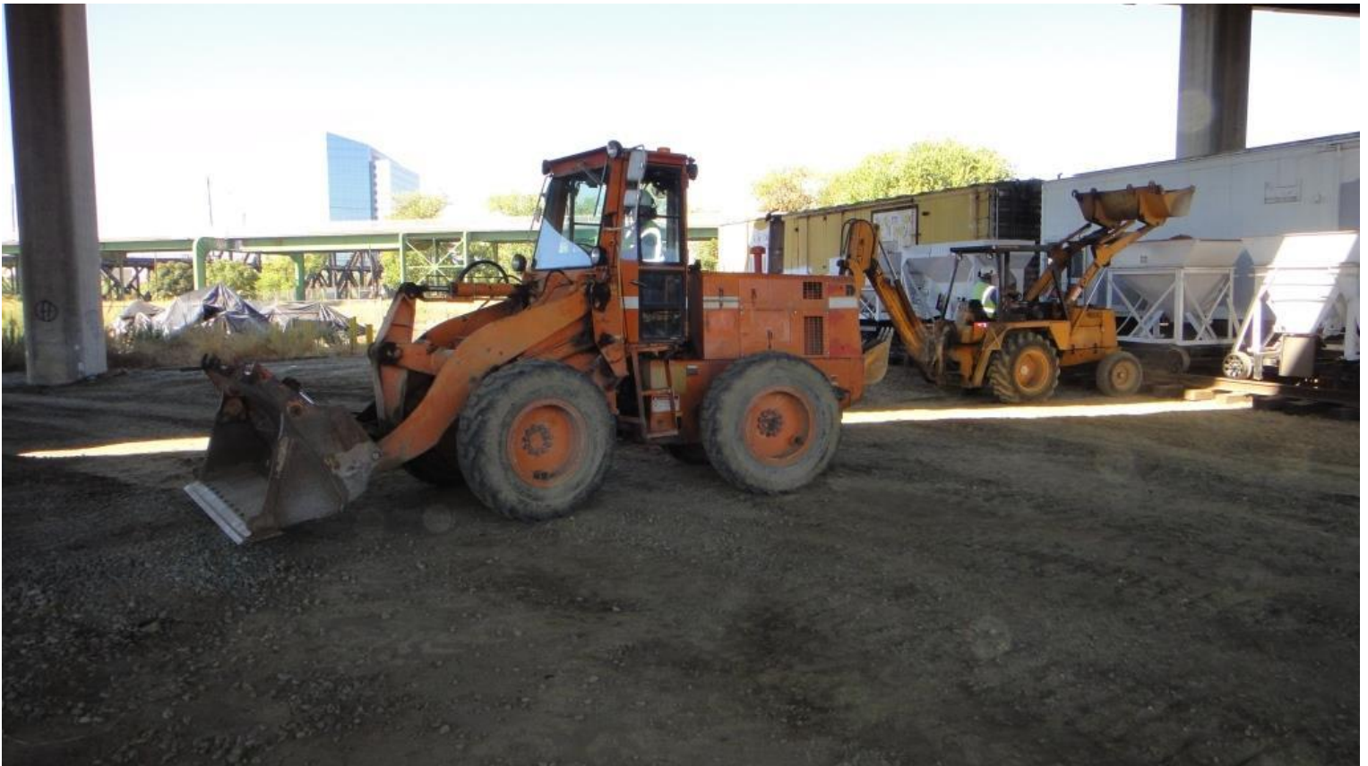
Steve in the front-end loader and Frank W. on the back-hoe load more rock and debris into the ballast cars
