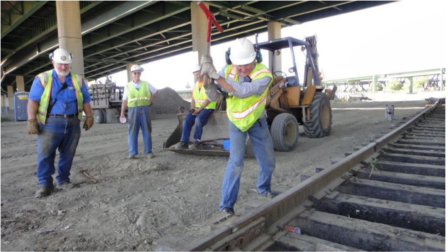
Steve demonstrates his world-famous "as seen on TV" patented windmill spike-driving technique
