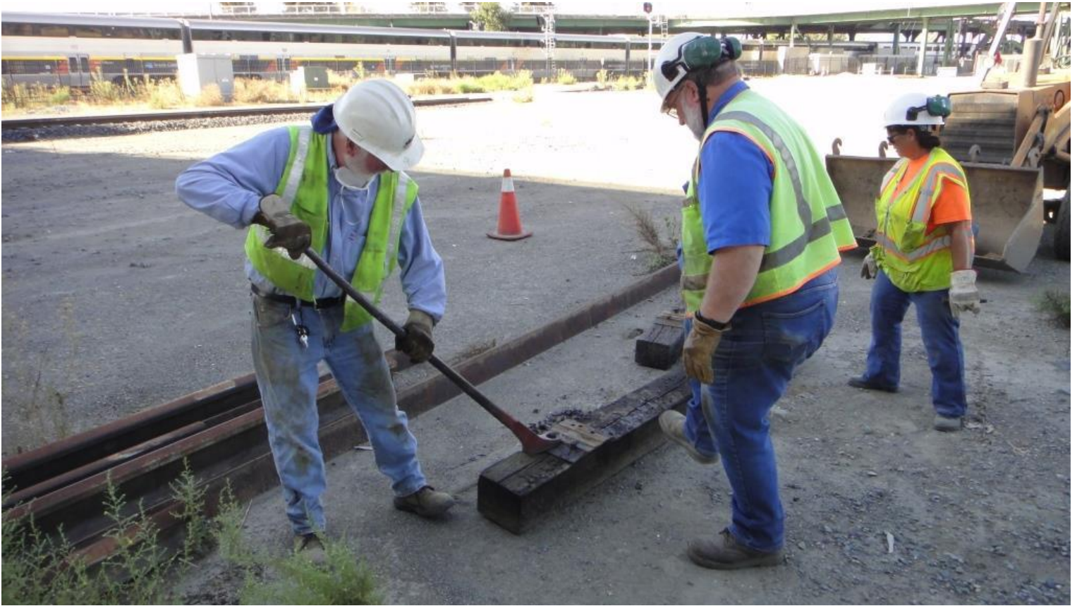
Robbing Peter to pay Paul – Mike M., Frank W., and Pam “steal” tie plates from the remaining segments of panel track
