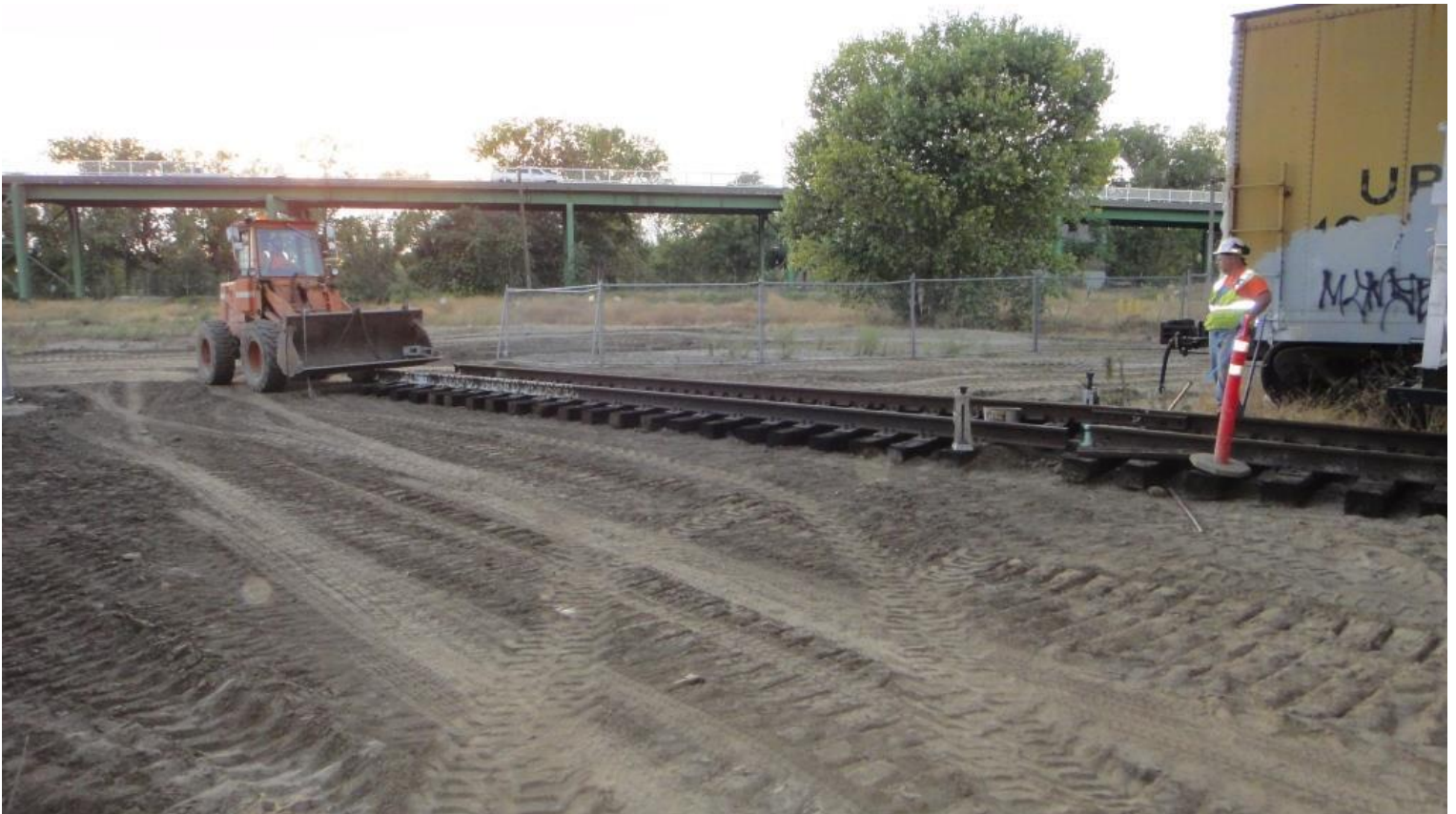
Under the direction of Mike F. on the ground, Frank W., in the front-end loader gives the track a little shove
