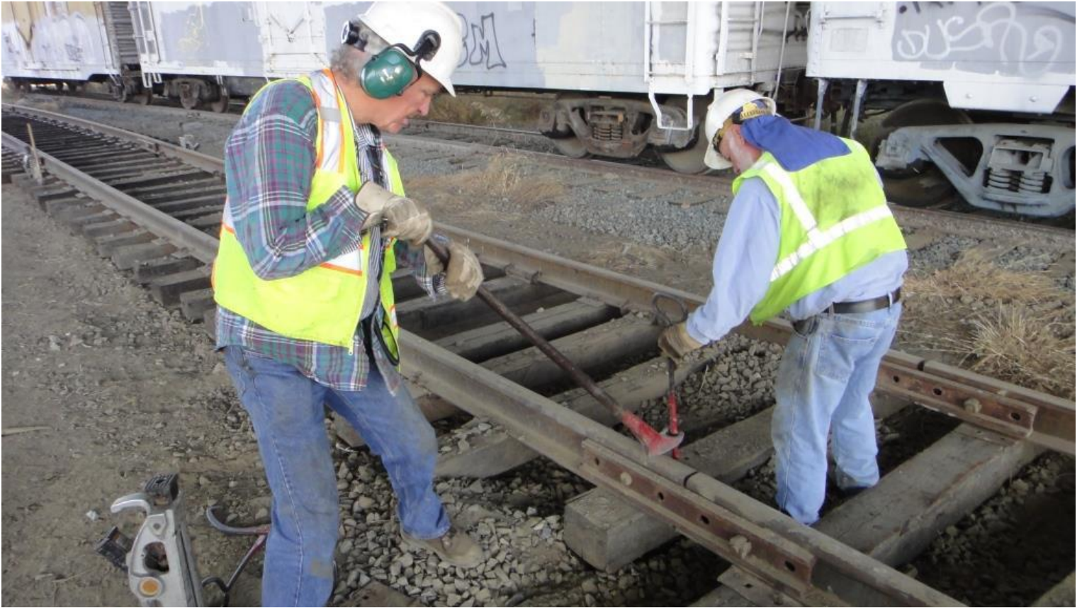
Steve and Mike M. use the claw-bar and "road-master" to pull a wayward spike
