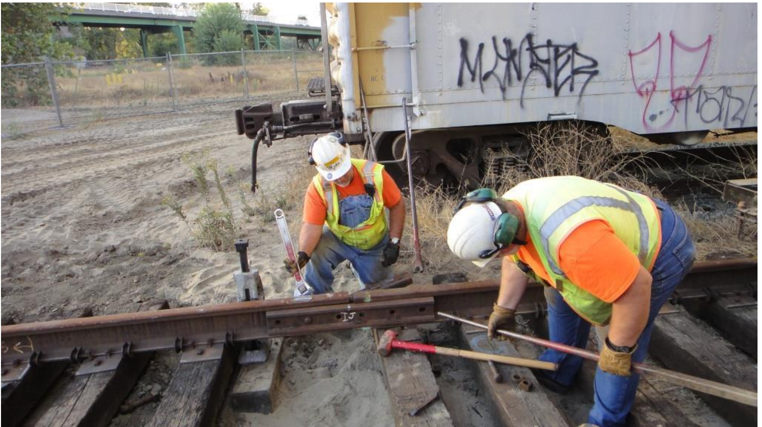
Mike F. and Frank W. line up the bolt-holes with the joint-bars
